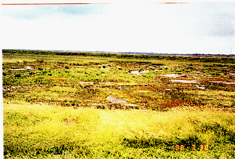
Figure 2.4 Horsey Island beneficial use of dredgings scheme. Lush vegetation had developed over part of the site within three months of the placement of the dredged material (Section 2.2.7).
