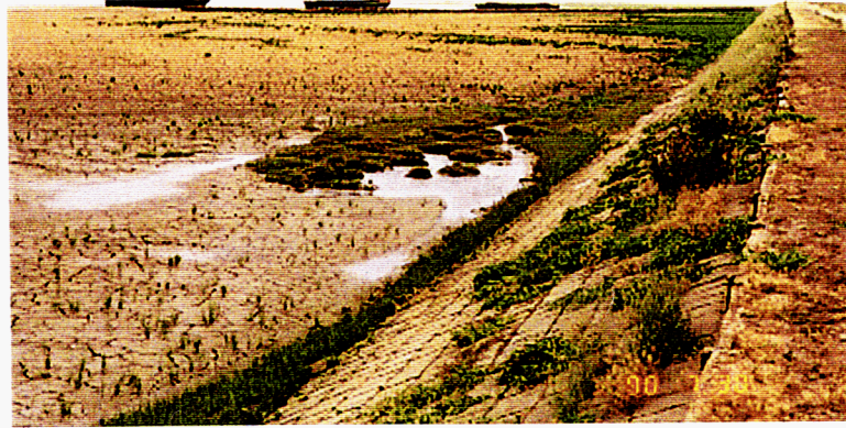
Figure 2.4 Horsey Island beneficial use of dredgings scheme. Lush vegetation had developed over part of the site within three months of the placement of the dredged material (Section 2.2.7).
