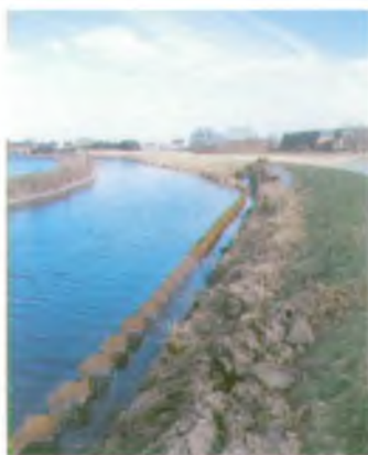
Sensitive Improvement Works – during construction
