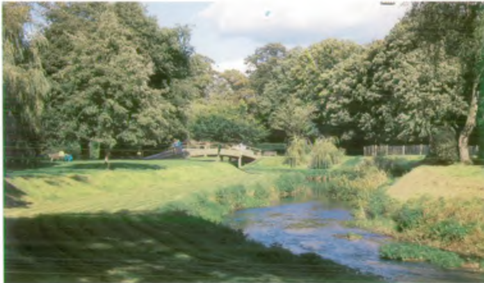
Capital works: landscaped 2 stage channel
