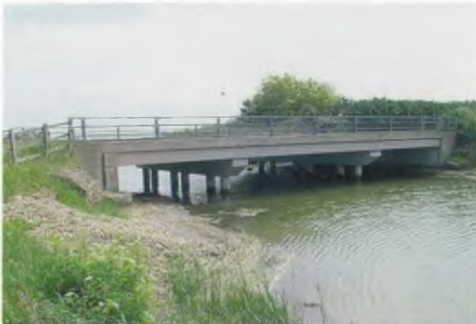
Photo 3 – A12 road bridge
