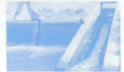
Automatic weir and fish pass
