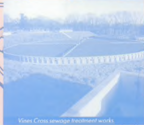
Vines Cross sewage treatment works
