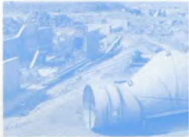
Installing the Hydro-Brake at the Aldington flood alleviation reservoir.
