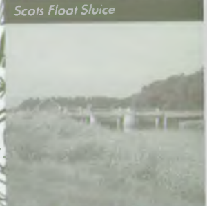
Scots Float Sluice
