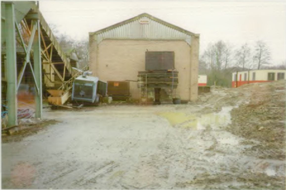
EXAMPLE OF TYPICAL UNBUNDED OIL TANK
