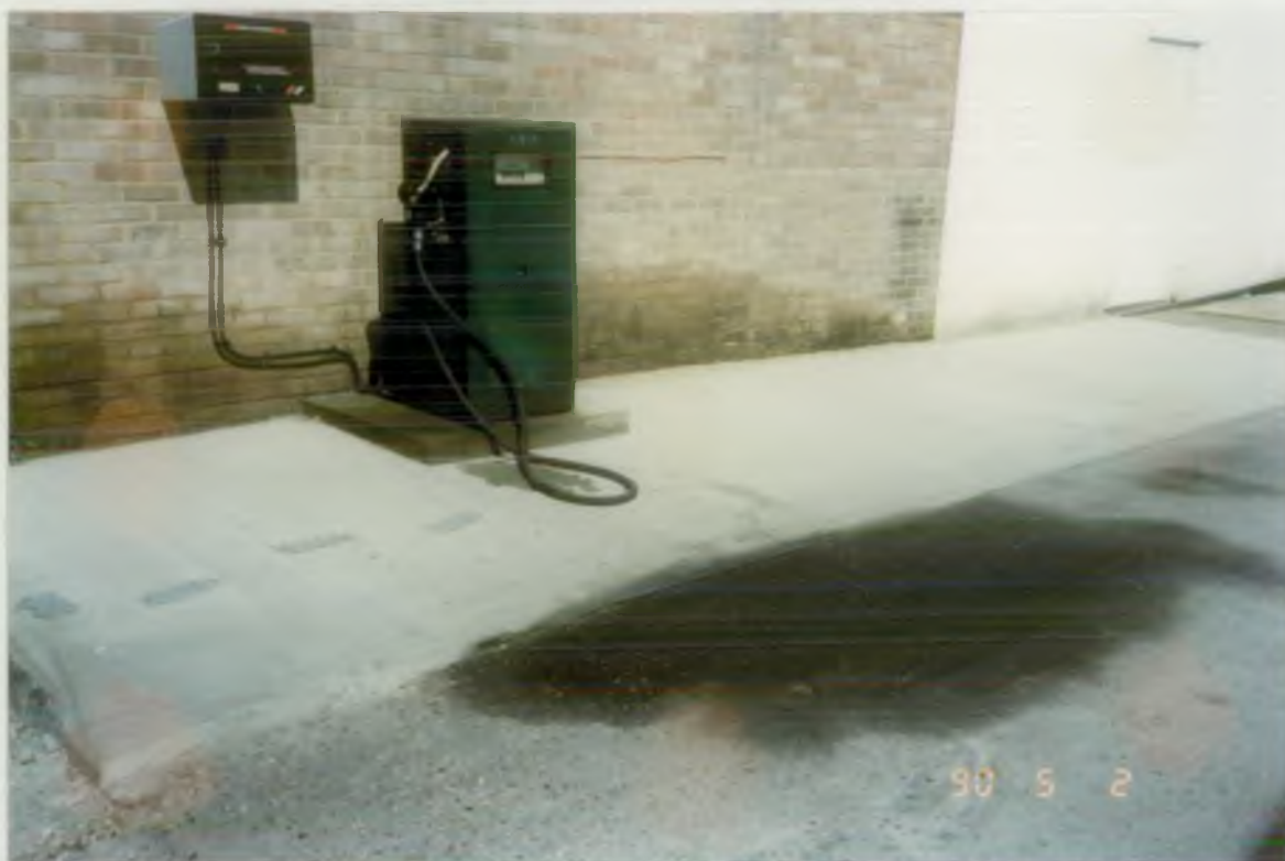
EXAMPLE OF A REFUELLING POINT
