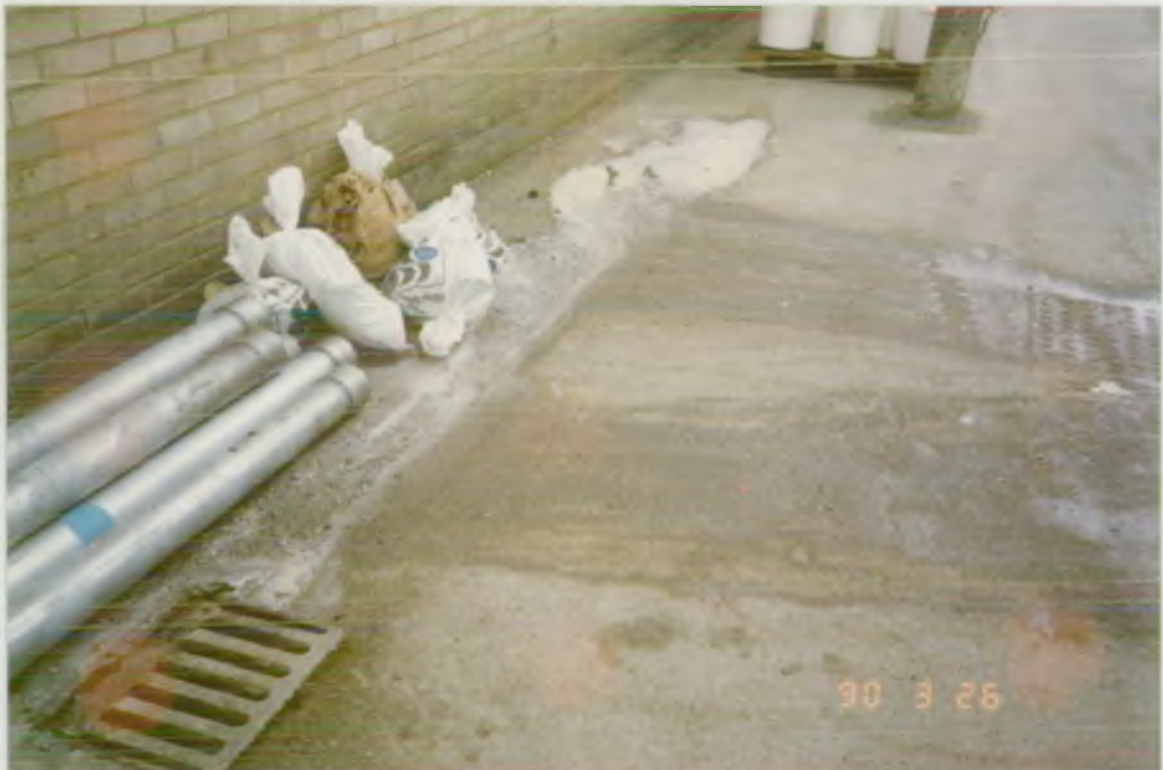
POLLUTION TO SURFACE WATER GULLEY AT FACTORY
