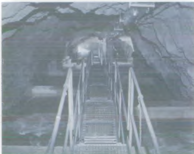
Inside the new Conwy falls fish pass.
