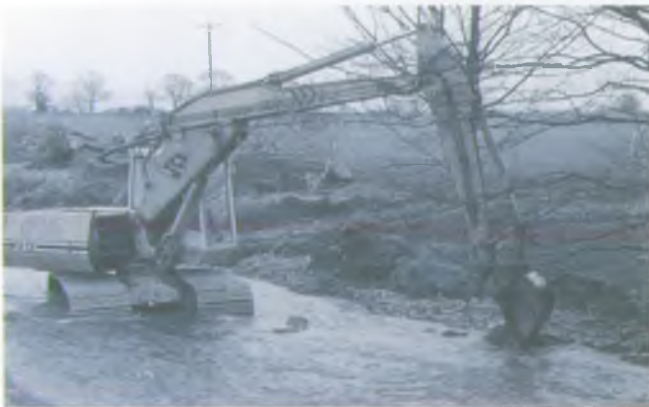
Flood defence work in the catchment
