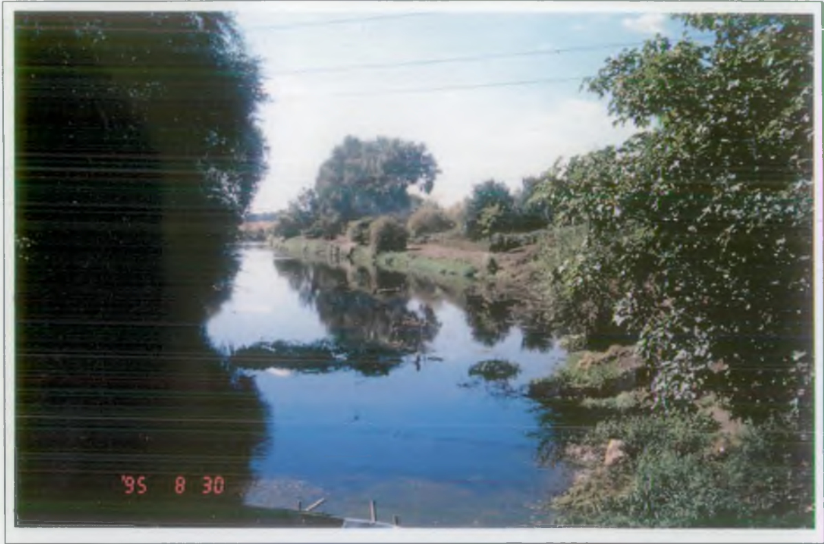
Start of work on 30 August 1995 - prior to dewatering
