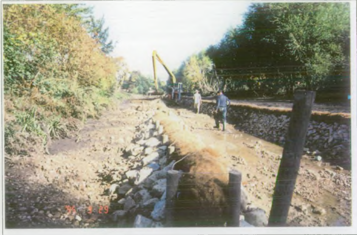
New low flow channel nearly complete, 29 September 1995
