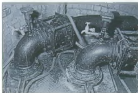
The top of a public supply borehole
