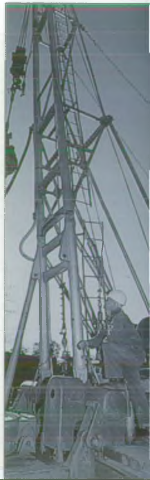
Drilling rig engaged in borehole construction
