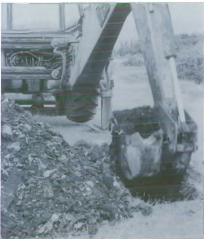
Trial pit investigation at a contaminated land site
