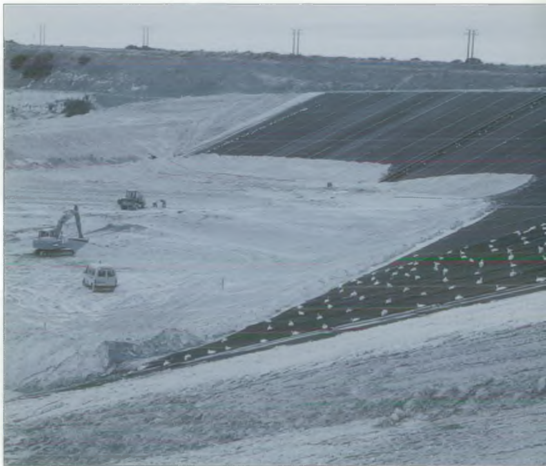
The lining of a new landfill on the Chalk with an artificial membrane in order to protect groundwater
