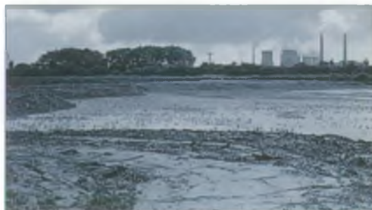
Pulverised fuel ash from power stations is deposited in sand and gravel excavations in the Trent valley
