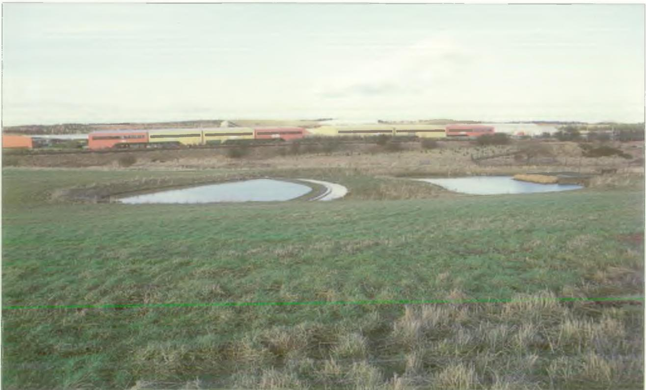
*This picture shows a filter strip that has been integrated into the pond design. The gravel filter strip provides a rooting medium for plants between the two sections of the pond. This pond serves an industrial estate in Livingstone.*
