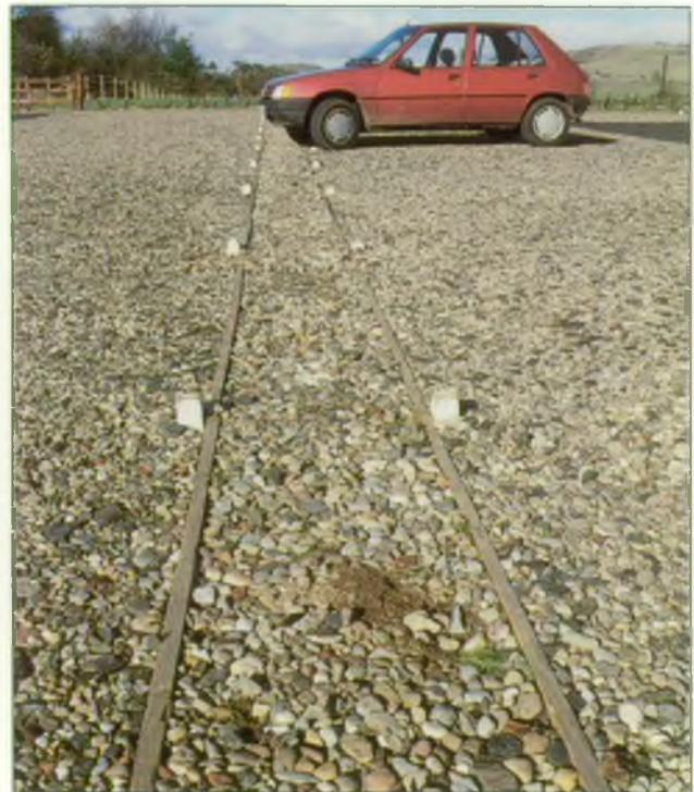
*This gravel car park area in Fife has an infiltration trench in the centre. Water soaks into the ground, but during high rainfall, the overflow pipe takes excess flow from the trench to a nearby stream.*
