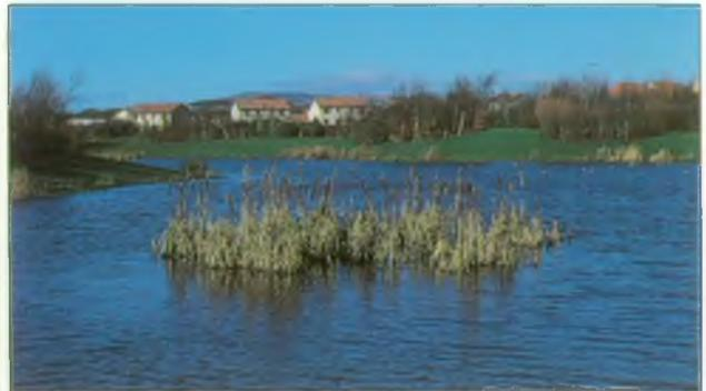
*Stenton Ponds in Glenrothes acts as both a flood control system and a water treatment pond.*
