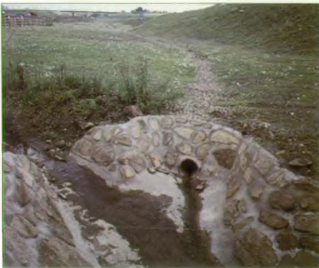
*This infiltration trench is incorporated into the landscape areas on a road embankment. The trench has an overflow into a stream.*
