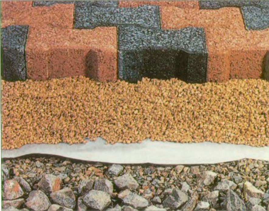
*UK manufactured porous blocks, being laid on a bed of ground and crushed stone. Porous surfaces are particularly appropriate for lightly contaminated runoff, close to source. The underlying materials provide a useful storage volume for peak storm events, for new or existing developments.*
