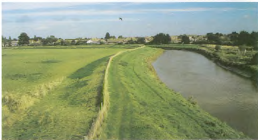
River Adur tidal embankments at Beeding
