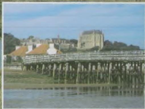
Alder Toll Bridge and Lancing College
