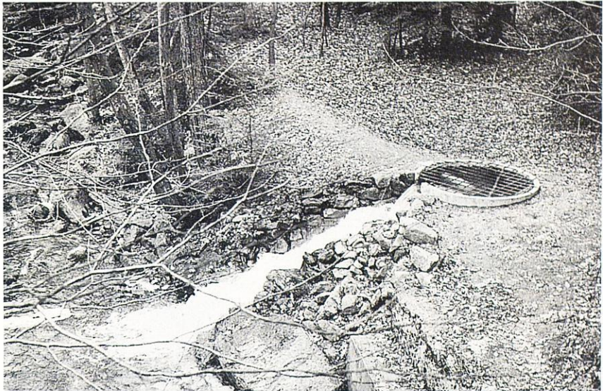
The Stony Creek diversion well, Pennsylvania, U.S.A.
